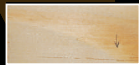
04 Seasoning checks / Grieta
